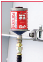
MB01-S bracket with BC30 beam clamp
